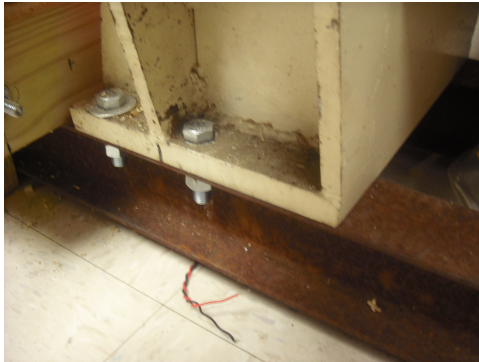
FIGURE B.4: Robot was bolted to steel I-beams from a Durham scrapyard.
