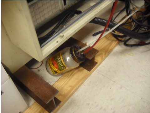
FIGURE B.12: Vacuum manifold. $2
